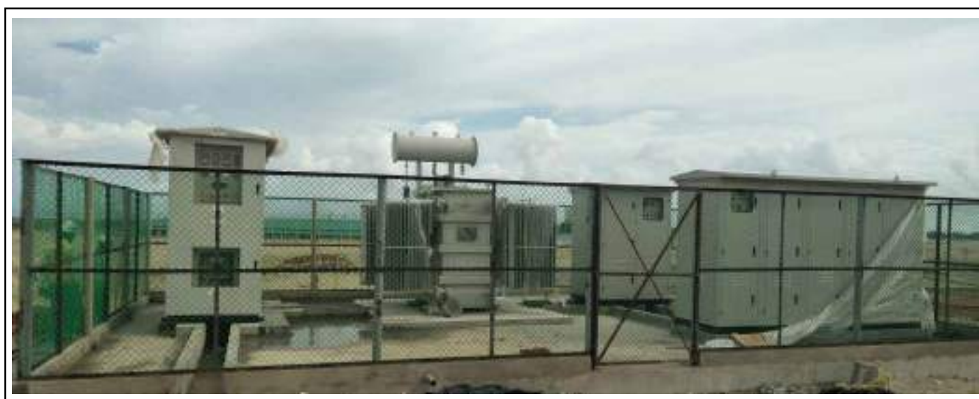
(Indoor VCB's in Outdoor use in 1250 MW Matarbari Coal-Fired Power Plant)
